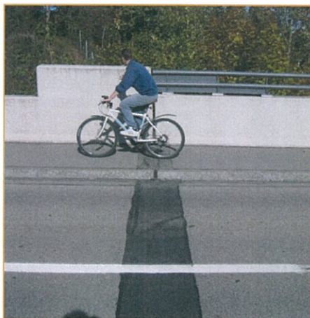
Original asphalt expansion joint
